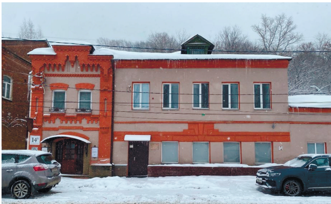
Pic. 3. Chernigovskaya street 14a and 14b
