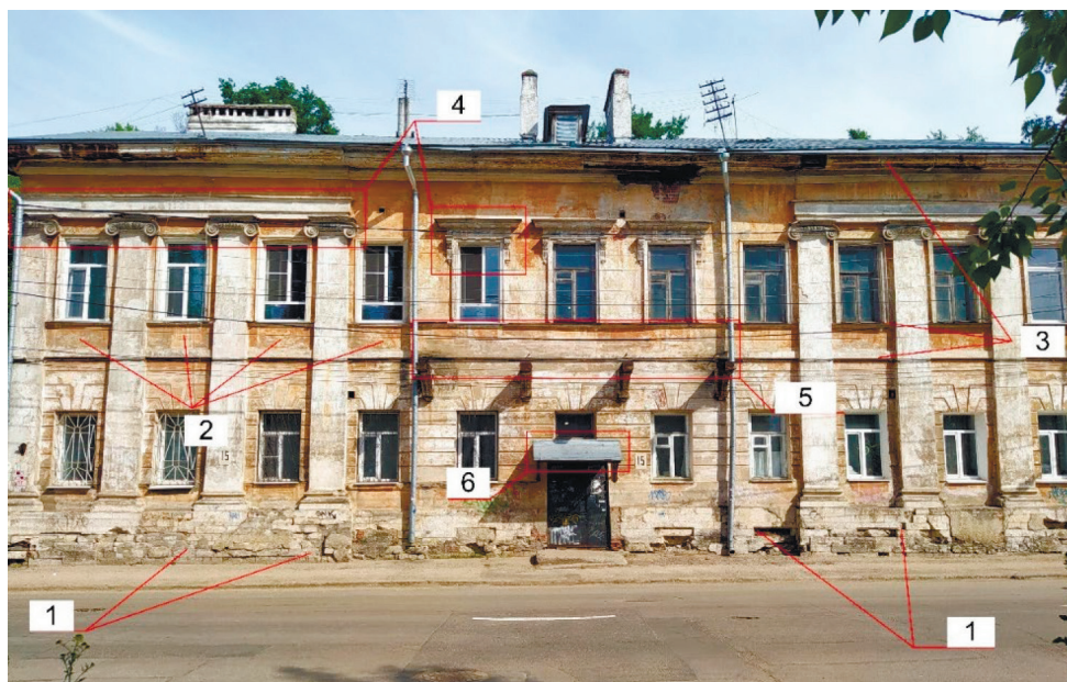
Pic. 6. Restoration of the Nenyukovs' house
